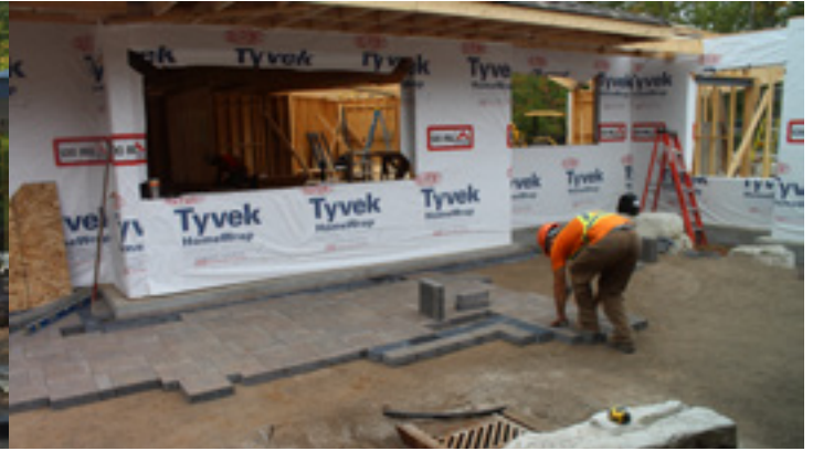
WEEK 14 | SEPT 18-22 Bricks are laid and walls are ready to be covered.
